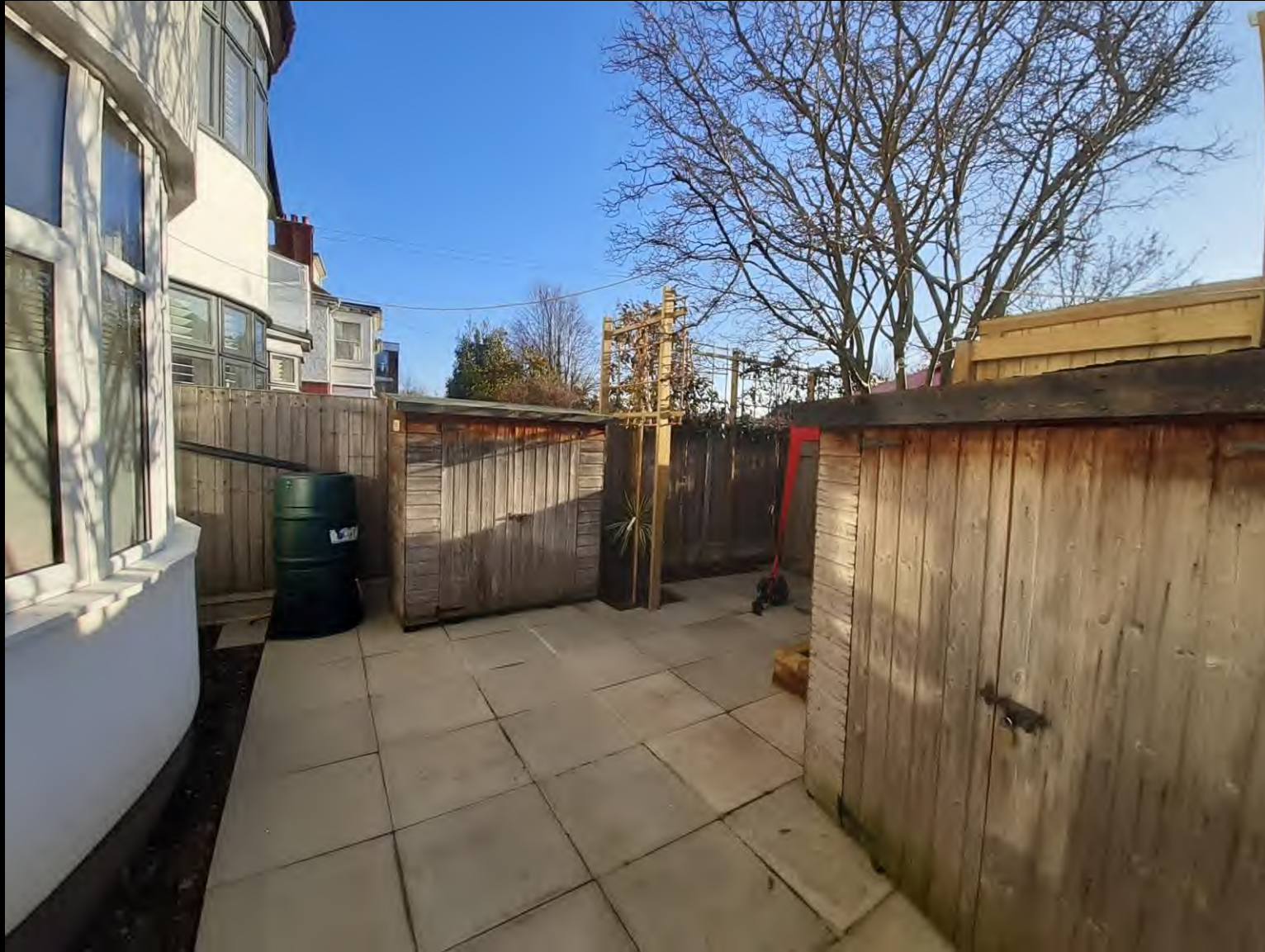
Enclosed area. Sheds are used for storage of prams, maintenance equipment and paraphernalia associated with nursery. Constrc. Manager advised that outbuildings have been on the front part of the site historically.
